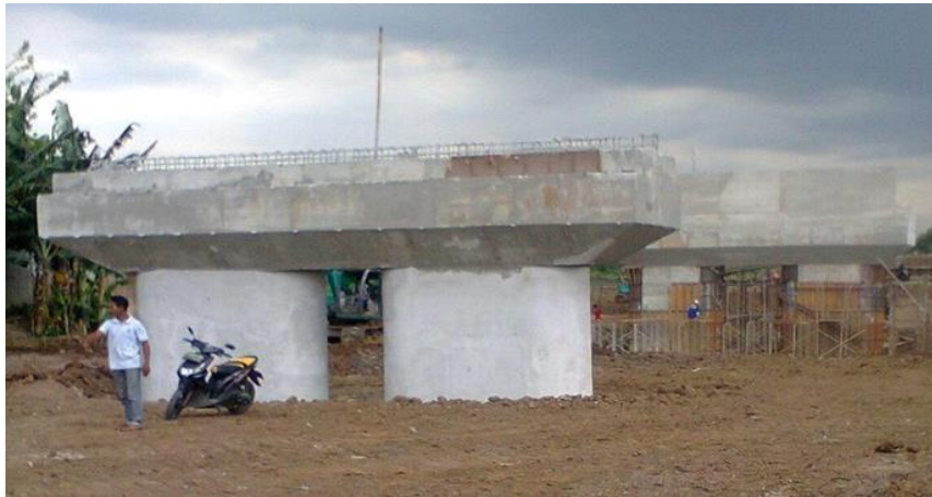
Gambar 3. 3 Pier Head Jembatan
